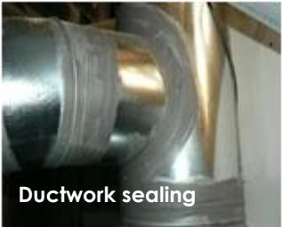
unheated/unconditioned part of the house, such as an unheated attic or garage. The test results should be listed on the energy component label. Supply ducts located outside of the conditioned part of the house must be insulated to at least R-8 and return ducts to at least R-6.
