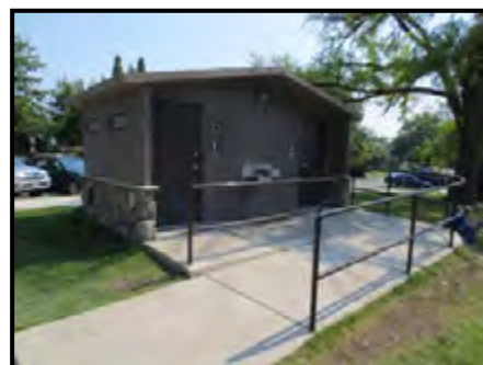
Baker Park Restrooms
