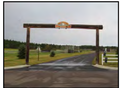
East entry area
