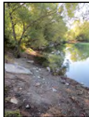
Informal river access and eroding banks
