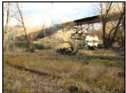
The BNSF train trestle over the Whitefish River at Skye Park
